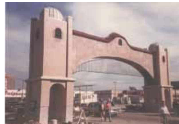
The Arch in the raw stage, standing just as beautiful completed.
